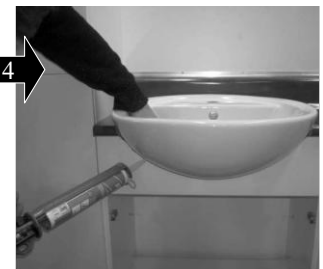
4 Apply silicone seal to front fascia
