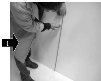
1 Determine the finished height
