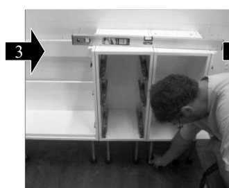
3 Screw feet down to the floor
