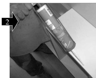
2 Make a suitable silicone seal onto the front of the unit
