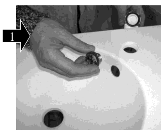
1 Install the overflow provided (it is advisable to fit the tap immediately after this step)
