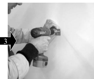
3 Fix the first wall plate
