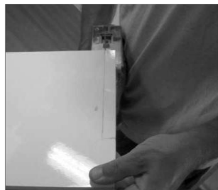
4 Where bath panel is fitted front plinth will have to be cut as shown above.
