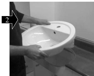
2 Fix basin into worktop with manufacturers brackets or silicone
