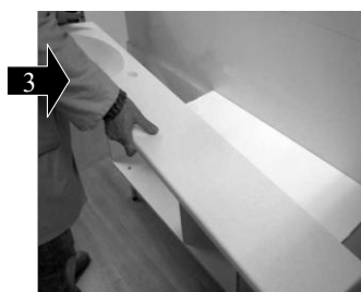
3 Position the worktop onto the units
