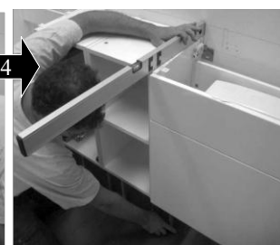
4 Adjust front to back levels
