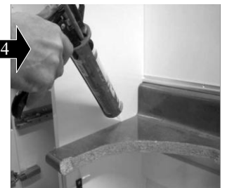
4 Apply silicone seal to all worktop edges including underside to carcass
