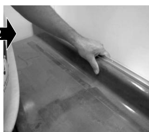
2 Position the worktop on the unit and against the wall
