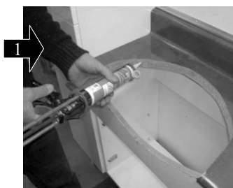
1 Apply silicone sealant to raw worktop edge to seal
