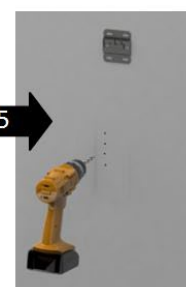
5 Drill the holes (screws and wall plug not provided)
