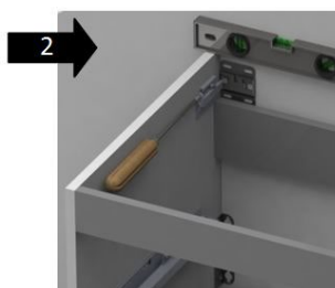
2 Tighten the brackets on the unit so that the furniture fits to the wall and adjust the levels
