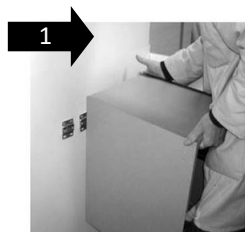
1 Hang the unit onto the wall plates
