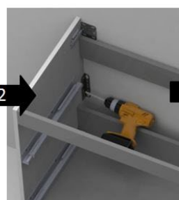
2 Fixing the brackets on the unit
