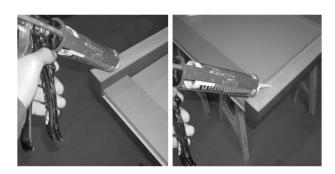
We recommended a silicone spot on each rear  $\underline{\text{bottom corner of the}}$   $\underline{\text{mirror}}$
