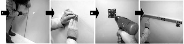
**1** Determine the finished height **2** Position the wall plate (see figure), mark and drill
