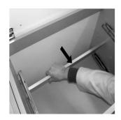
APPLY A SMALL AMOUNT OF SILICONE ON THE FRONT TOP OF THE UNITS
