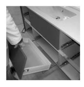
Make sure the unit is level so that adjusting is not too difficult
